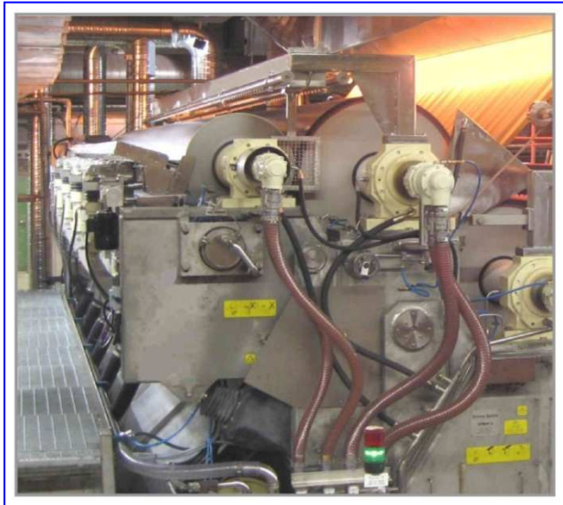
Fig. 12 Foto TWIN™Sizer, Gravure coater(MONO) installed at Korsnäs Frövi Board mill
